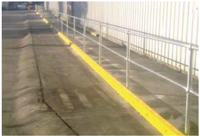
Asset and pedestrian protection.
